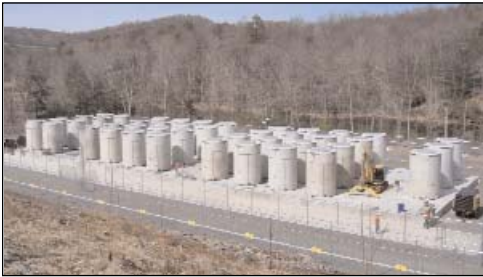
Connecticut Yankee Fuel Storage Facility
