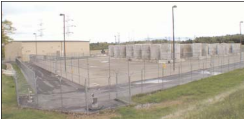
Maine Yankee Fuel Storage Facility
