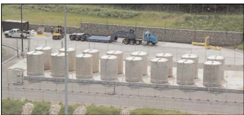
Yankee Rowe Fuel Storage Facility
